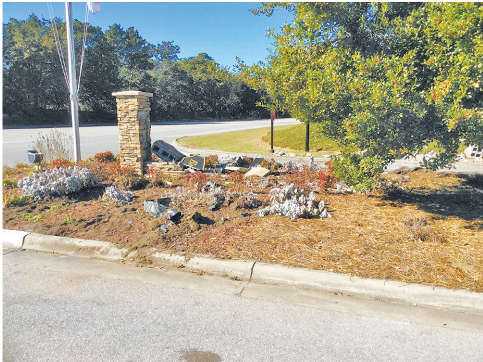
Hwy 24 Sign Damage: The entrance sign for the golf side of Brandywine Bay on Hwy. 24 was damaged on January 24, 2018 in a single-car accident. Thankfully, there were no injuries due to the accident. The BOA Board is working with the car's insurance company to replace the signage back to the original design. Thank you for your patience as we clean up the area. Photo submitted by Bob Workman.
